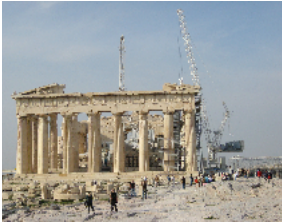
Even when built to last, care is needed.
